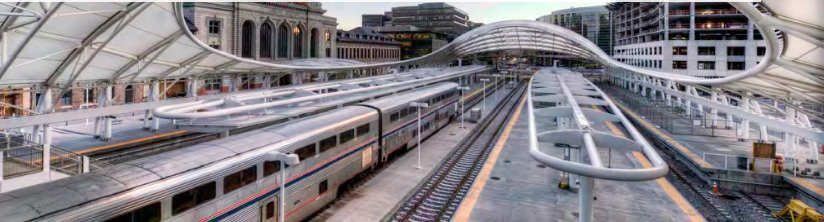
Denver Union Station Transit Improvements (Image Source: Design-Build Institute of America)
