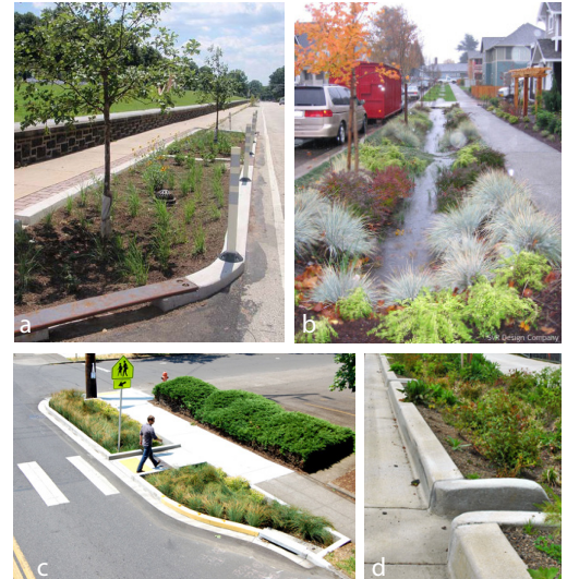
Examples of natural drainage strategies that support stormwater and walkability: a) curb extension, b) planted swale, c) curb extension with crosswalk, d) curb and gutter detail shows curb cut that allows stormwater to flow into planted swale.
