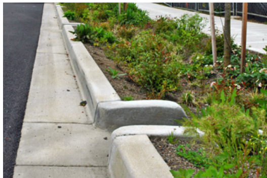
Example of a curb cut that allows stormwater from street gutter to flow into a planted swale.
