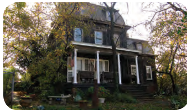
Located on Richmond Terrace and designated as a landmark site, the John De Groot House is an example of historic architecture located close to industrial uses.
