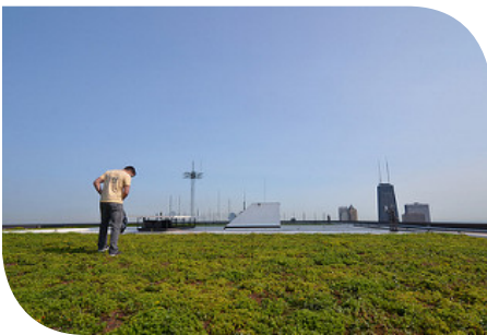
Replacing black asphalt roofs with green roofs reduces peak temperature by up to 60 degrees and reduces winter heat loss by 34 percent, saving residents money.
