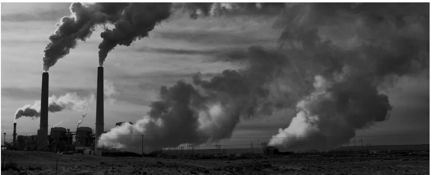
Cholla Power Plant in Arizona (Magnus Manske) (Source: commons.wikimedia.org/wiki/File:Cholla_power_plant.jpg)
