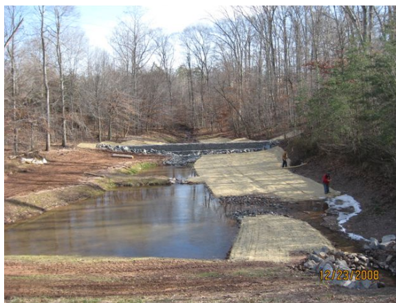
Above: Before (top) and after (bottom) photos of Compton Heights regional stormwater pond retrofit project.
