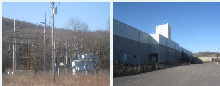
Electric substation (left); Building 5 (right); Warehouse (bottom)
