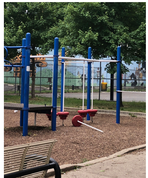
Broken playground equipment at Edgewood Avenue Playground.
