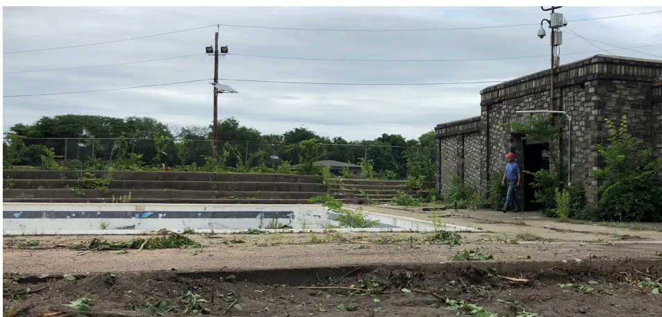
Renovations are underway at the historic Hetzel pool facility.
