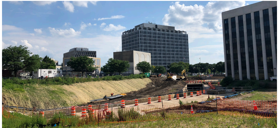
Daylighting of the Assunpink Creek in downtown Trenton.
