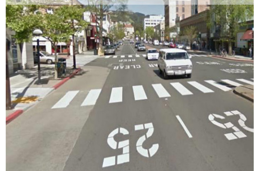
The University Avenue repaving project added High Visibility Crosswalk markings and Advance Stop Bars to improve pedestrian visibility and safety.
