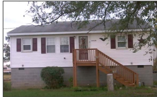
Figure 1. Home where neighbors report no indoor plumbing.
