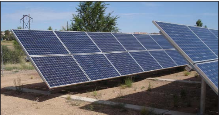
Solar photovoltaic (PV) panels
