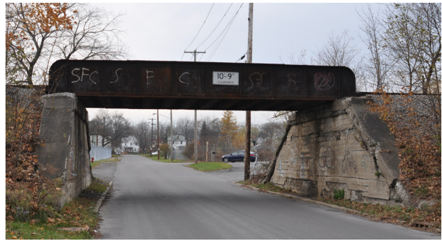
Railroad underpass at Gates Avenue
