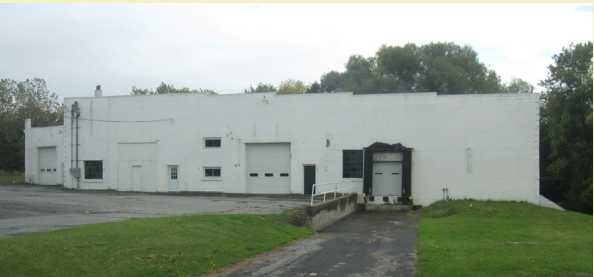
Structures on Wadsworth Street (top) and Avenue B (right) show varied housing quality; commercial buildings on Exchange Street (middle) and Middle Street (bottom).
