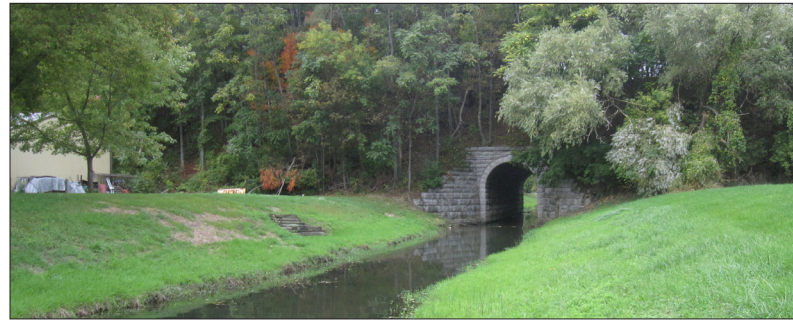
Marsh Creek and tunnel under the inactive elevated rail line.
