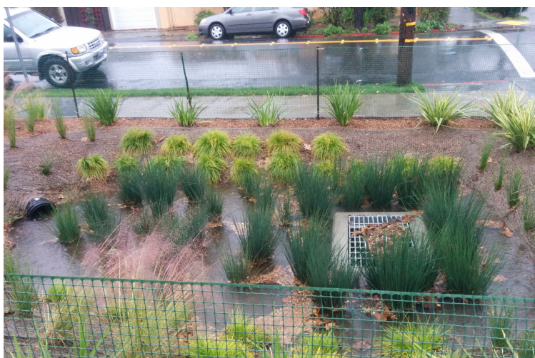
Directing stormwater runoff into rain gardens or bioswales reduces street flooding and allows stormwater to infiltrate rather than enter the storm drain network.
