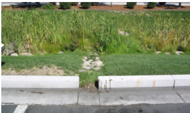
Curb cuts provide a path for flooding water to move away from streets and sidewalks. In some situations, curb cuts can be created retroactively.
