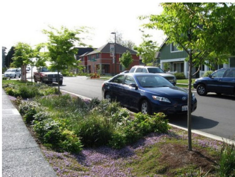
Swales that convey stormwater can be integrated with streets, sidewalks and bike lanes in neighborhoods and urban areas. Hardscapes such as streets and sidewalks can also be converted to pervious surfaces that help absorb rainwater.
