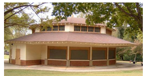
Original Carousel Building
